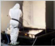
Indoor Foam Application
